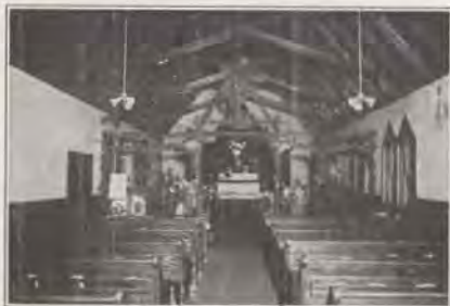
St. Luke's, Showing Open Rafters Before Fire
