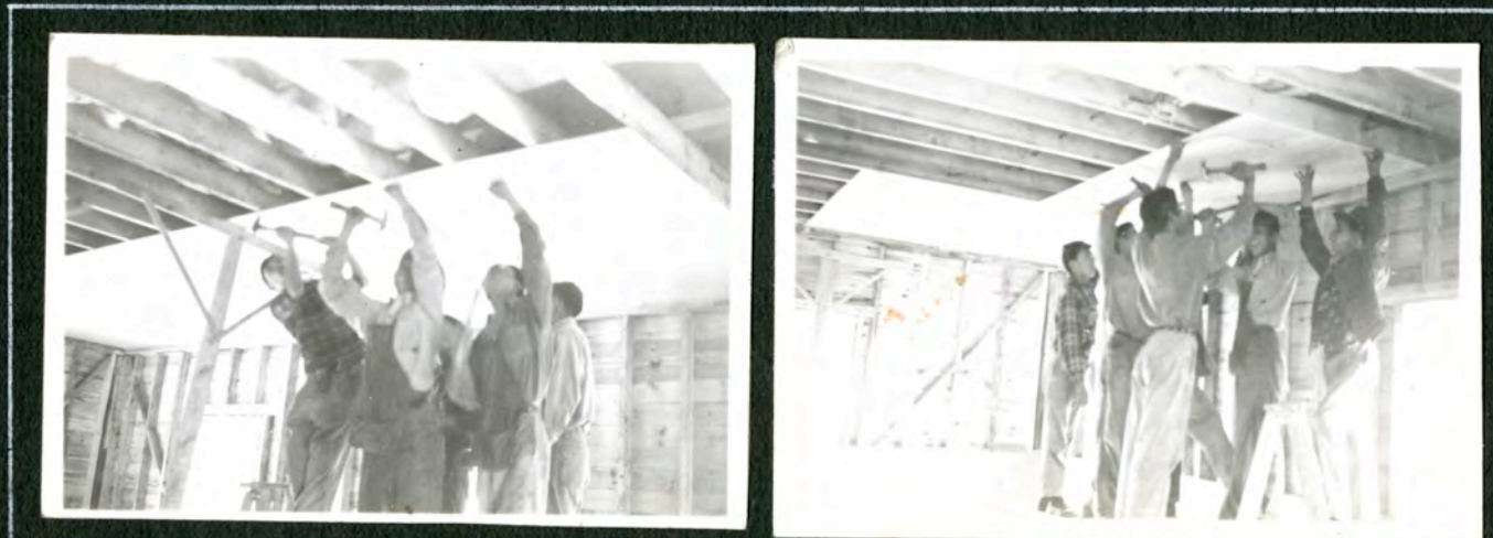
BOYS APPLYING GYPROC TO CEILING OF SHOP
