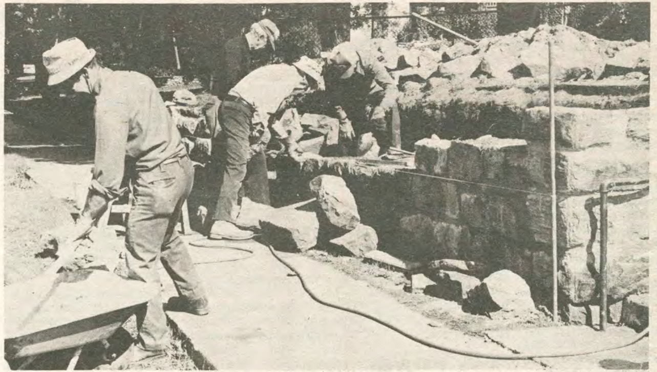
REBUILD TRINITY WALL: Volunteers from the Trinity Church congregation at Parry Sound had a busy time during the fall season rebuilding the stone wall in front of the church. They used most of the original stones from the wall which it is believed was about 75 years old. The volunteers were, left to right, Bernard
