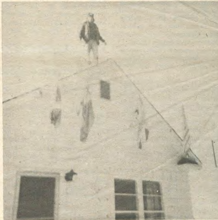
SNOW AND ICE CLEARING: As described in the accompanying article, after helping clear off the roof of the rectory at Dorset, Randy Curnow found a quick way to descend by jumping.
