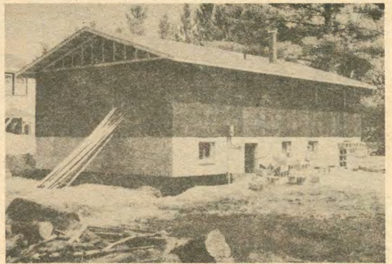
Here is a picture of the New Residence under construction at the Society of St. John the Evangelist in Bracebridge, Ontario. This picture was taken this summer.
