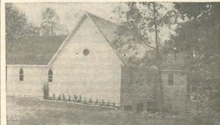
Above, St. Mark's Church, Milford Bay, showing new vestry on left.
