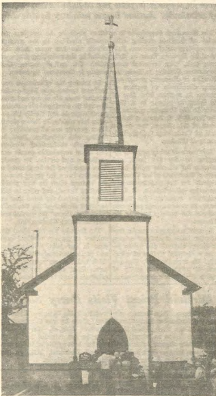
St. Paul's Church, Manitowaning
