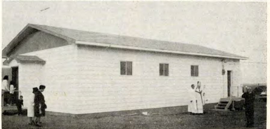
The erection of the new St. Anthony's mission chapel, near Griswold, Manitoba, was made possible through the co-operation of the Oblate Fathers who provided lay and scholastic Brothers for its construction, of the K of C of St. Lazare council who donated labor, the parishioners of Dunrea and the Ladies' Auxiliary of Birtle. A substantial donation was also made by the diocese to supplement the insurance money received when the former chapel was destroyed by fire in 1964. Photos: Archbishop G. B. Flahiff blesses the new chapel; a former missionary Father G. Laviolette, preached in Dakota on that occasion.
