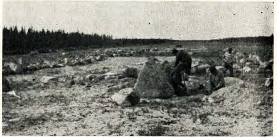
Landing strip in the making at Brochet, Alberta.
