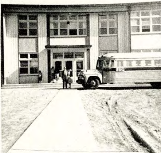
School Bus at main door
