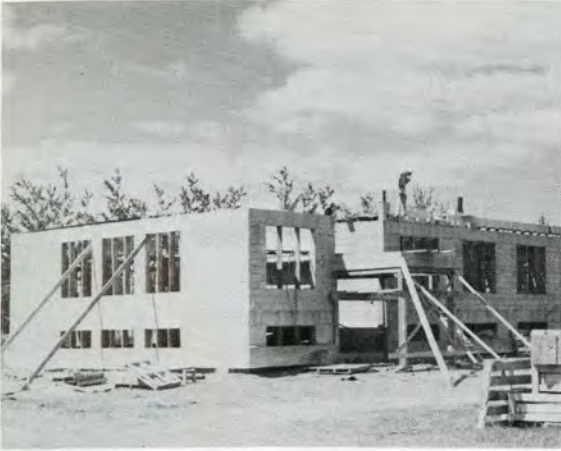
Building under construction
