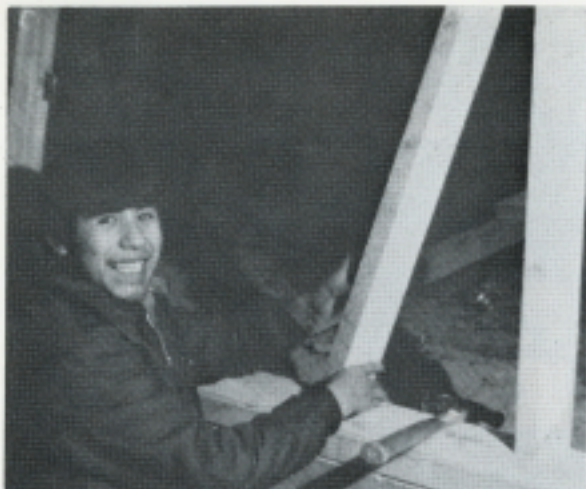
Nailing Studs
