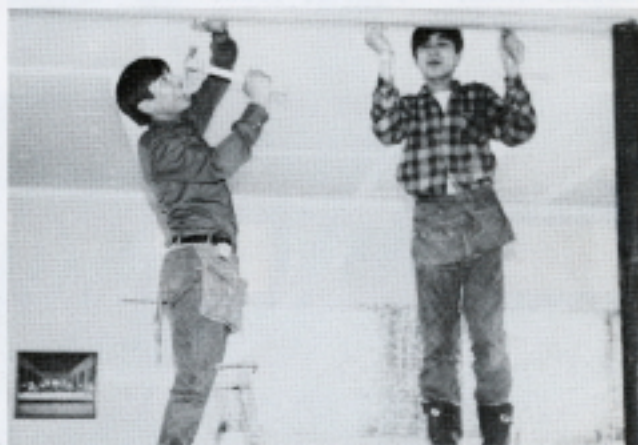
We hung drywall in our building project. We set our nails so that we could plaster over them. Allan
