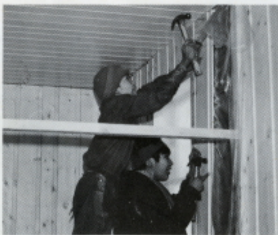
We put up the panelling. First we cut spruce boards with the table saw. Then we sanded them so they would be smooth. Allen
