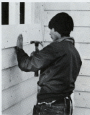
Nailing on the siding
