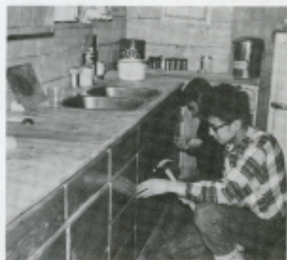
Finishing the set of cupboards
