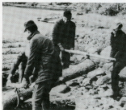
Pulling the logs to shore
