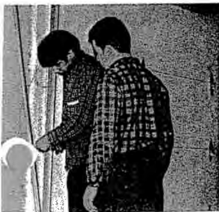
Installing overhead door
