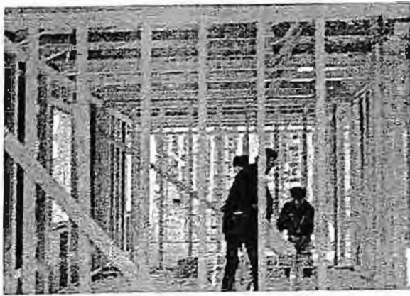
The framework of the new house.
