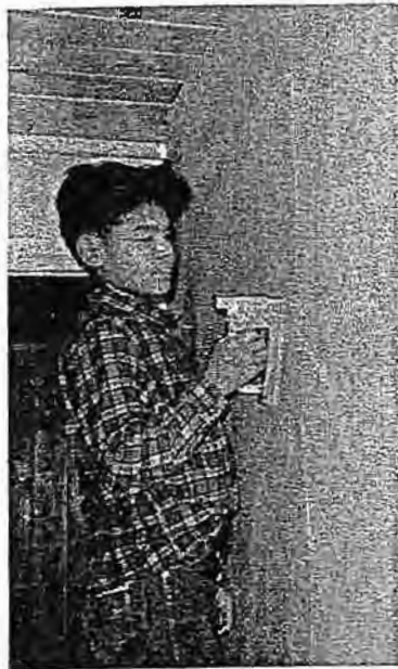
"We'll soon be ready for the wallpaper."
