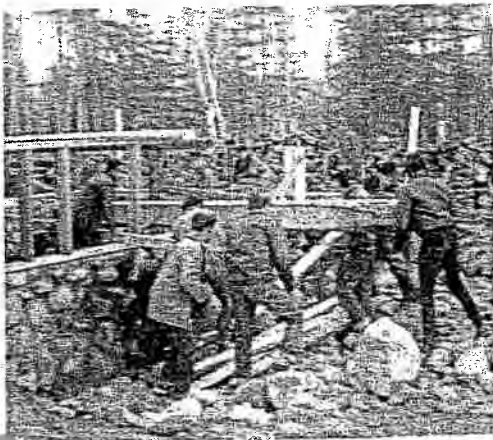
Placing and fitting a girder
