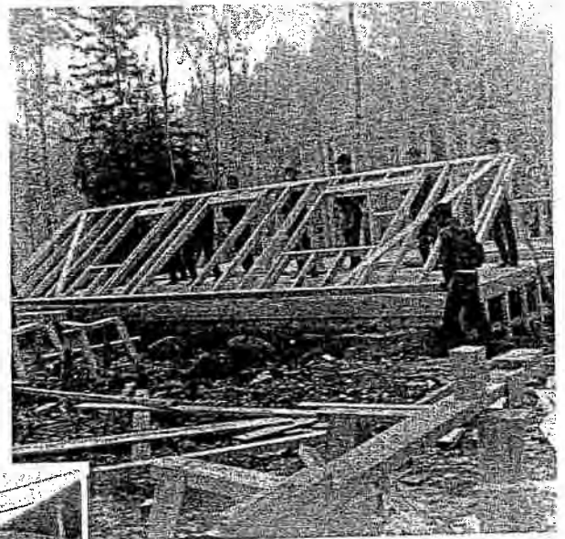
Lifting the framework
