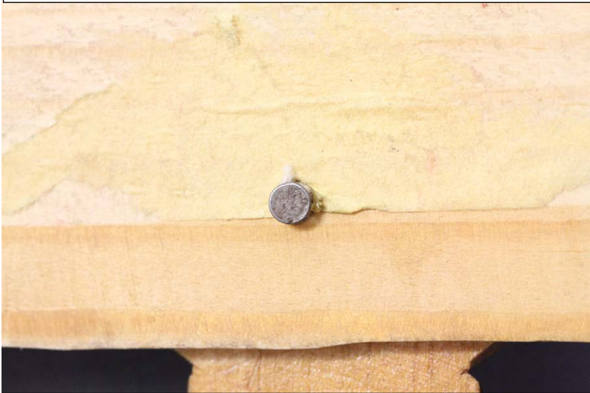
Fig.4 – Corrosion – Back center
