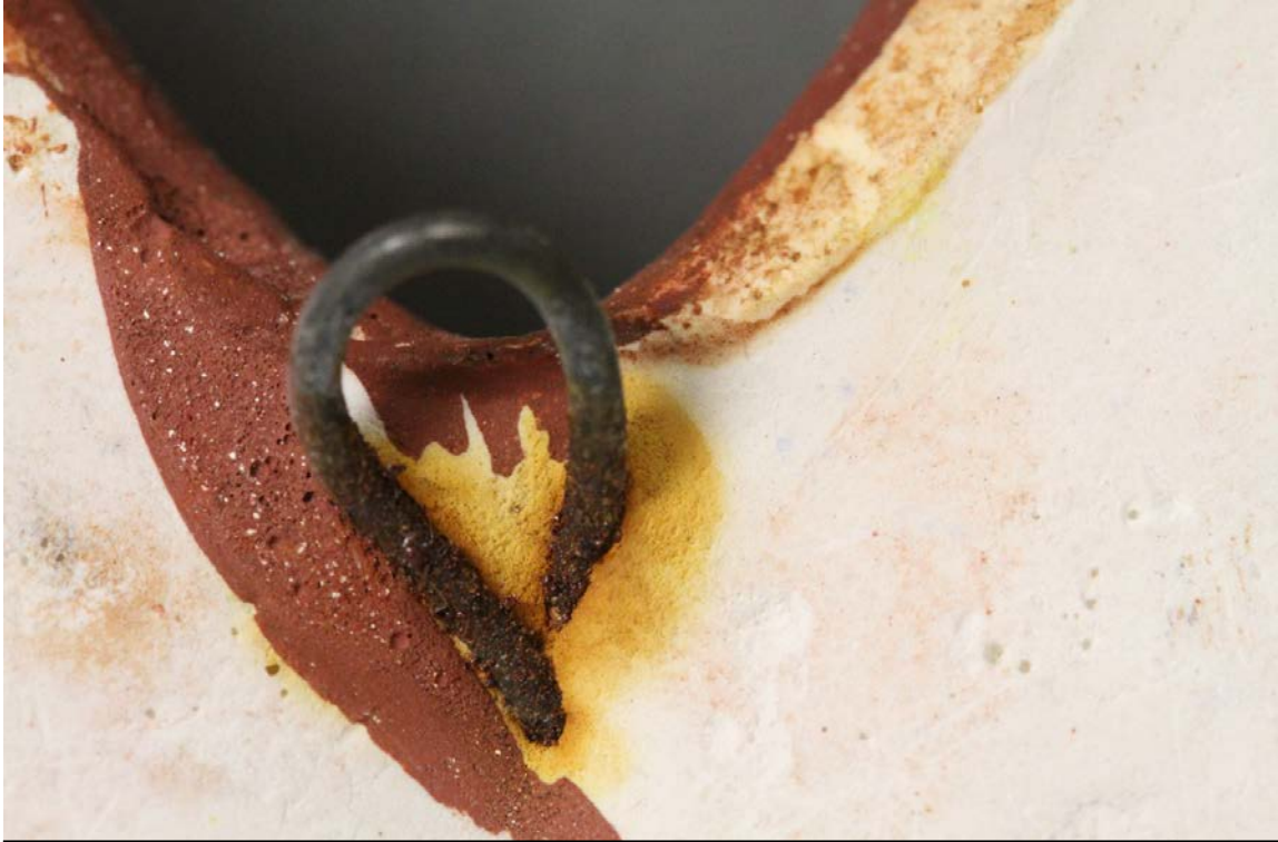
Fig.5 – Corrosion – Back top center
