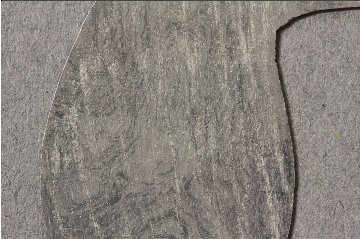
Fig.4 – Corrosion – Back center
