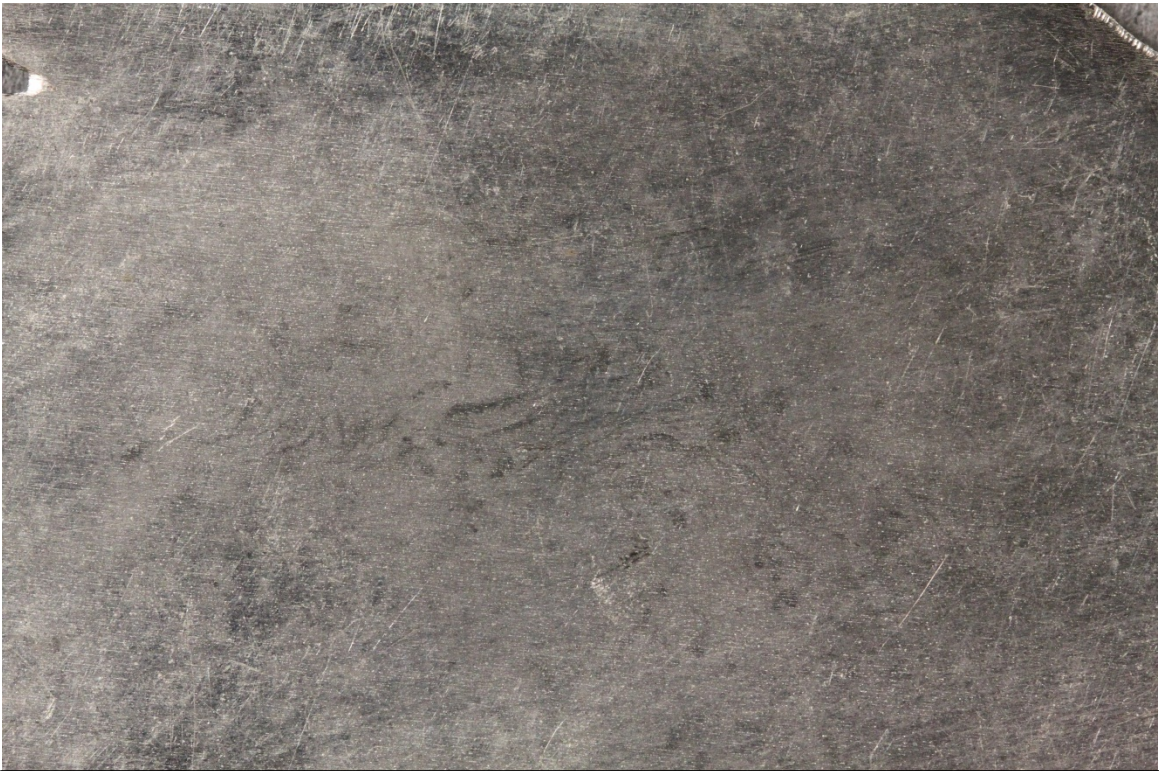
Fig.3 – Corrosion – Back center
