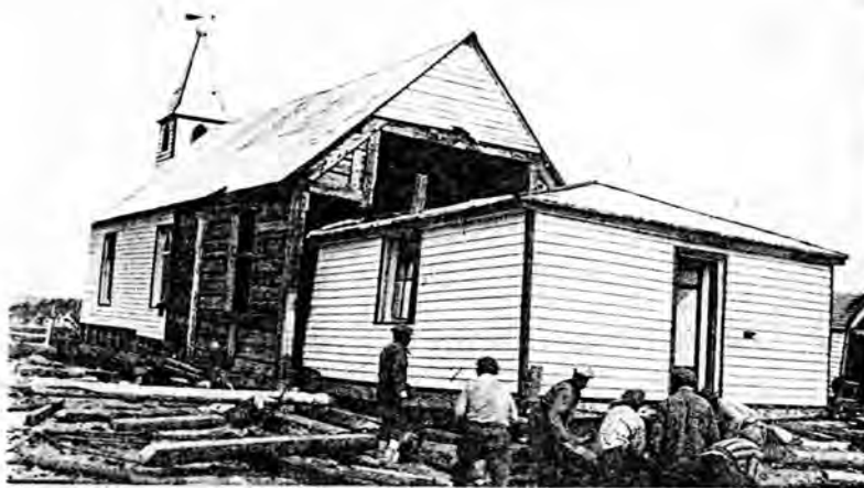
St. Philip's Church being reassembled after being moved to safer ground. The native men did much of the work.
