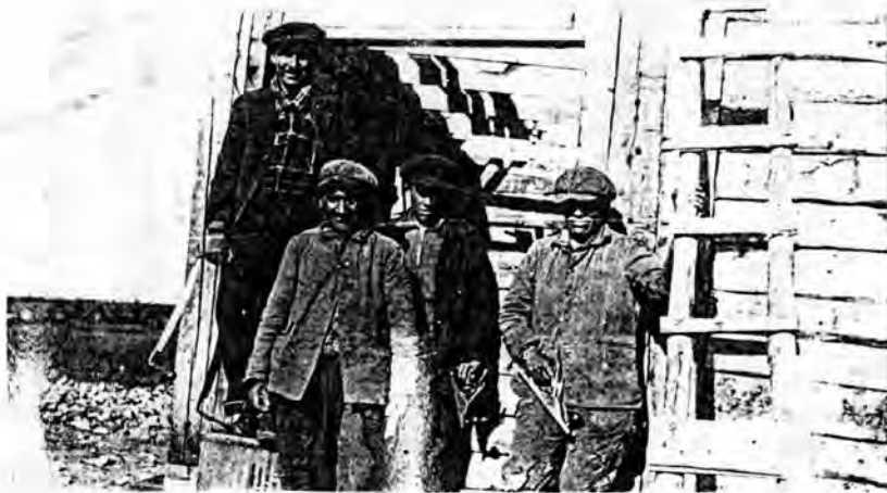
These men helped to build the residential school at Fort George. From left: Sam Iserhoff, Noah Kapisco, Sammy Linklighter, and an unidentified man.
