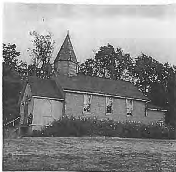
Wesley Church at its original location.
