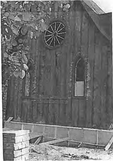
Much time and care has gone into restoring the historic community church as this picture indicates. courtesy of Harry Brown
