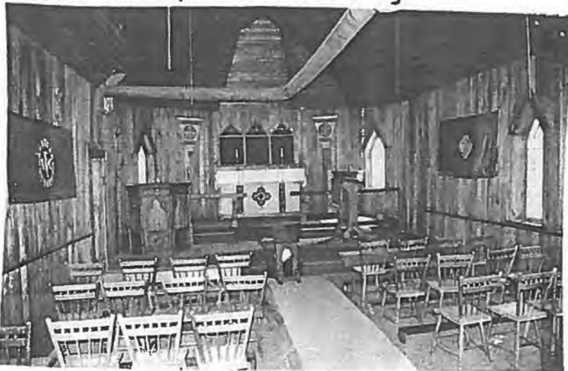
The interior of St. George's Church is relatively the same as it was in 1880 when the structure was built.
