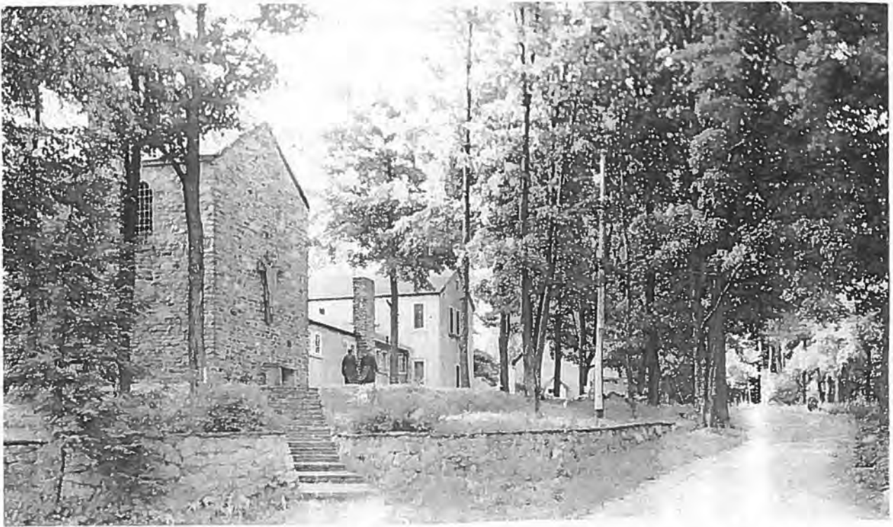
The S.S.J.E. Church and Mission House, Bracebridge.
