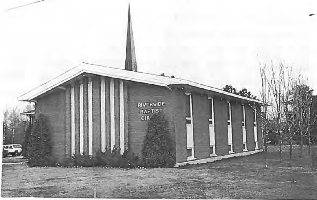
Riverside Baptist Church as of May 1, 1996.
